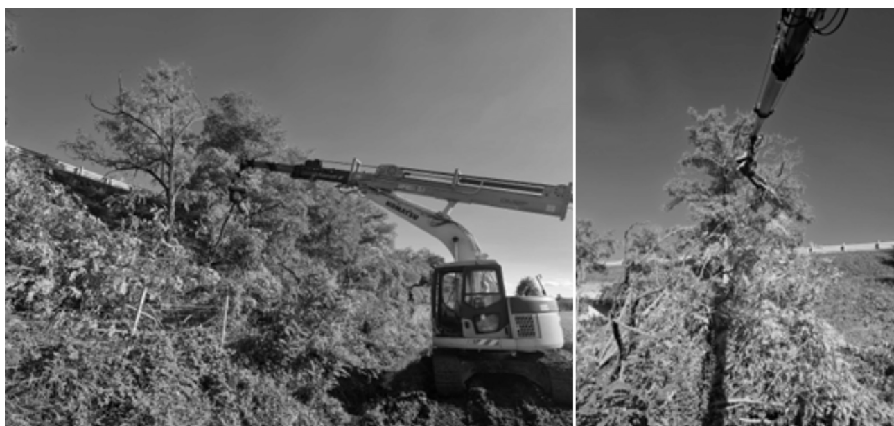
Fig. 5 Specific machine at work in highway embankment
