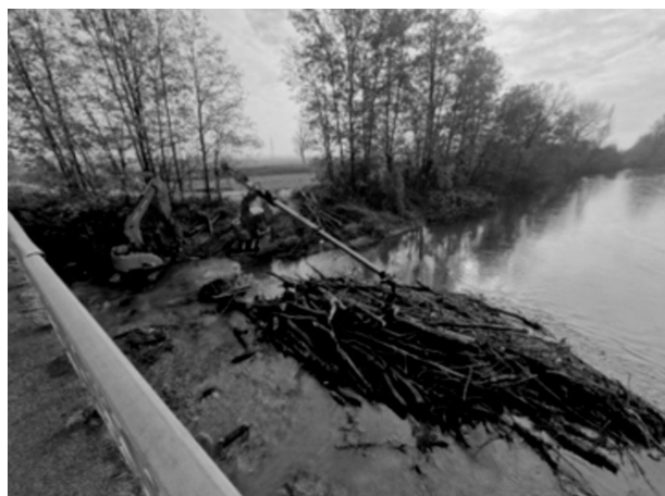
Fig. 10 Removal of logs near a bridge
