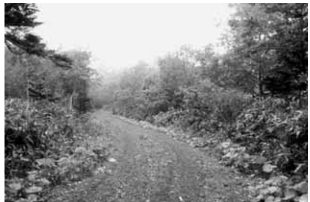
Figure 1 Well maintained main forest road (Maeyama, constructed in 1968. Base rock is welded tuff.)
