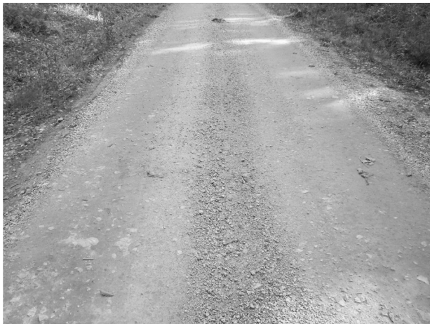
Fig. 14 Macadam pavement built on lime stabilization (Ver. 6)
