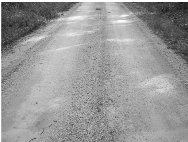
Fig. 15 Unsurfaced lime stabilization (Ver. 5)
