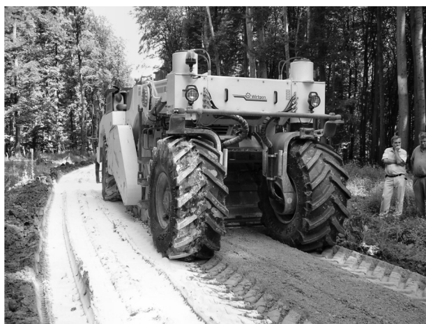
Fig. 3 Soil milling machine
