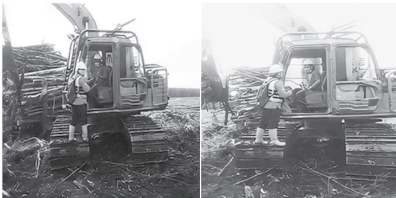
Fig. 3 Excavator Hitachi ZX110MF
